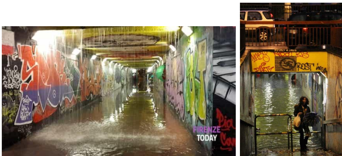
Figure 25 Flooding of the pedestrian underpass below the railway track and adjacent road junctions, October 2, 2016 (street level totally below the surrounding ground level).
